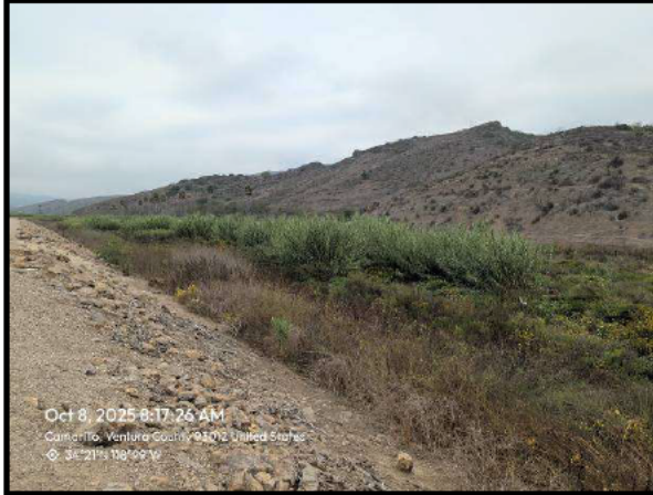
Looking upstream from western levee prior to Project activities, October 8, 2025.
