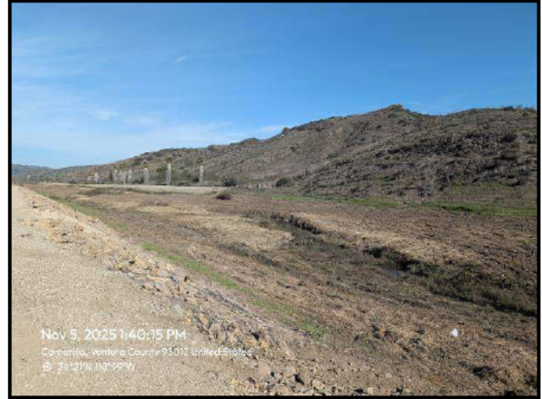
Looking upstream from western levee following Project activities, November 5, 2025.
