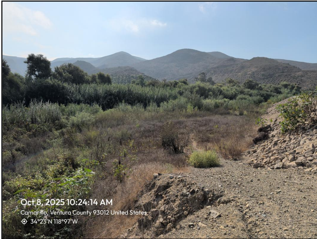
Photo 15. Looking downstream (southeast) from the west levee access Road near the confluence with Upland Road Drain prior to project activities, October 8, 2025.
