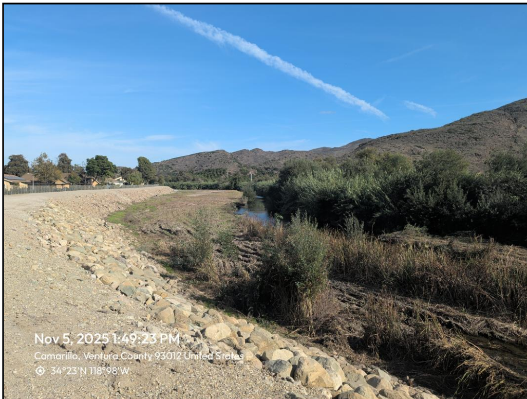
Photo 14. Looking upstream (east) from the west levee access road following project activities, November 5, 2025.
