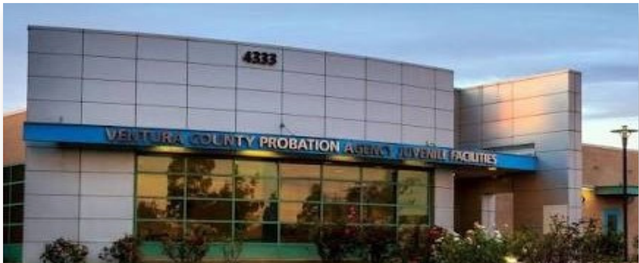
Ventura County's Juvenile Facility is part of the Juvenile Justice Center in Oxnard. (Photo courtesy of Ventura County Probation Agency)
