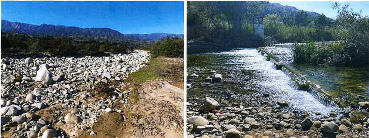
Figure 1. Typical examples of large cobbles and boulder substrates in the Ventura River and at the exposed portion of the subsurface dam, which are not appropriate materials for jet grouting.
