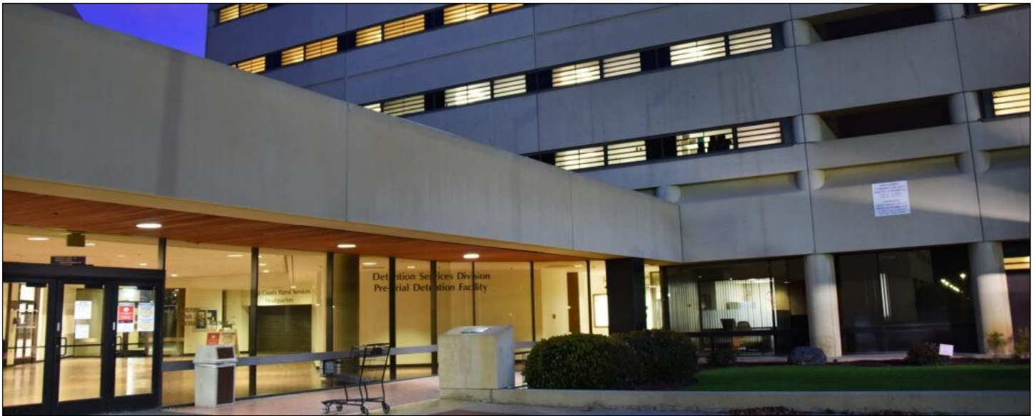
Entrance to the Pre-Trial Detention Facility (Main Jail) at the Ventura County Government Center. (Photo courtesy of Ventura County Sheriff Office)
